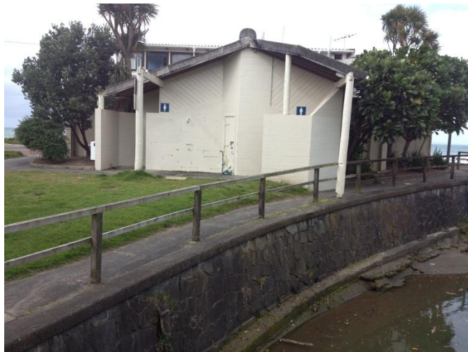
Public toilets adjacent to the surf club
