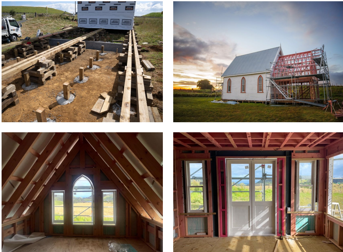
Fig. 41 Construction activity on the Kobekobe Church. Re-piling and new structure. Photographs courtesy of Guy Quartermain.
