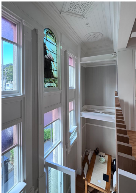
Fig. 60 Exterior and interior views of the newly transformed Esplanade Heights. The southwestern unit's design features a void in the former church's transept. Changes like a relocated ceiling fretwork panel in the main bedroom, and new skylight and south-facing window openings enhance natural light, ventilation, and adapt to the new internal layout. Photographs by Elisa Aguirre.
