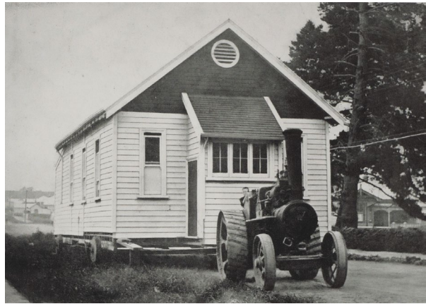
Fig. 19 A church is being towed by traction engine to a new site, in November 1911.
