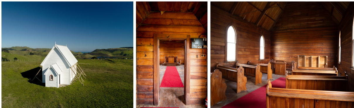
Fig. 40 The Kohekohe Church before its adaptive reuse. Temporary supports were placed to stabilise the building due to the imminent risk of collapse. Photographs courtesy of Guy Quartermain.
