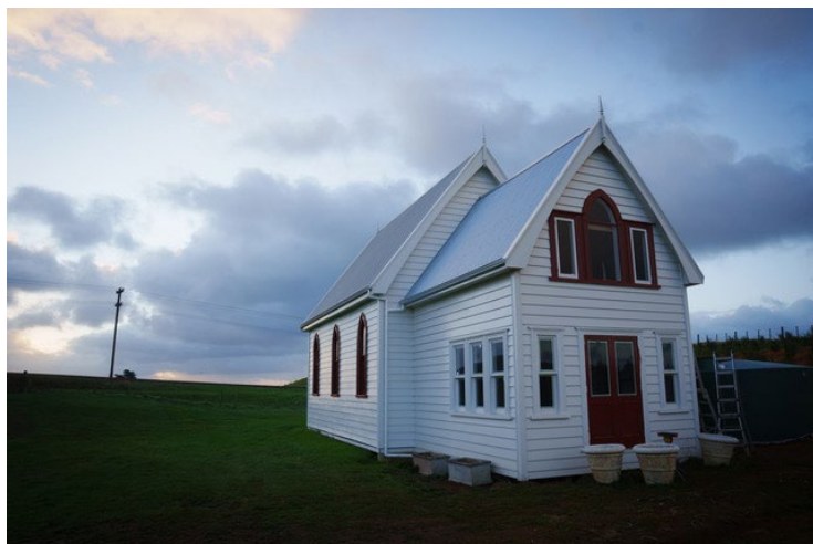
Fig. 43 Exterior views of the Kohekohe Church post-adaptation. The addition at the rear is largely concealed from the road due to its smaller scale and strategic positioning. Photographs courtesy of Guy Quartermain.
