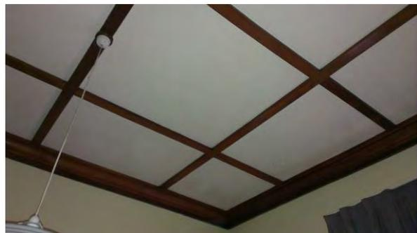
**Figure 6:** Timber batten ceiling (Auckland Council, 2013)
