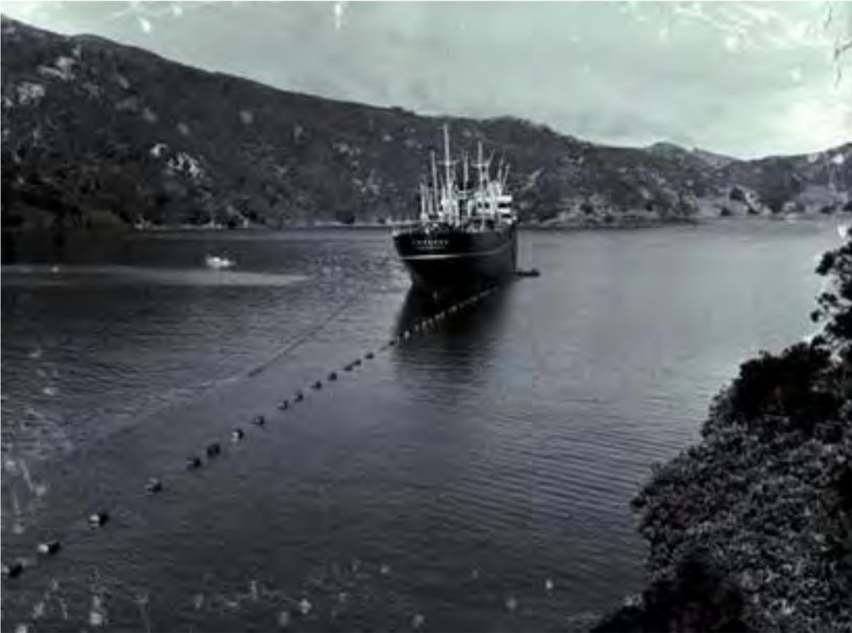
Figure 122. Whale oil being pumped to the vessel *Tiranna* in Whangaparapara Bay. The pipeline is supported by a combination of 44-gallon drums and reused harbour defence buoys. (AWMM/L PH-NEG-H51).
