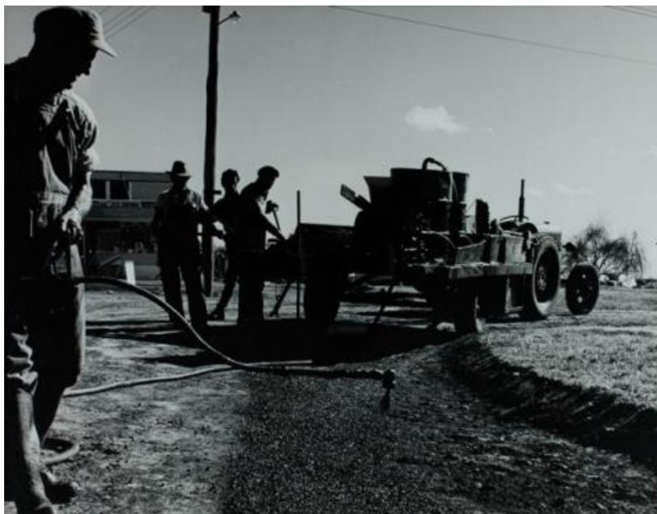
**Figure 66:** Papatoetoe Borough Council workmen spreading tar on a road, 1962. One of a series of photographs commissioned by Papatoetoe Borough Council during the town's centennial year. (Auckland Libraries Footprints 02571).
