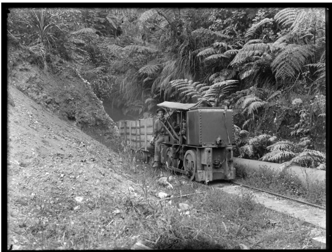
Nihotupu tramline and pipe route during construction of the Upper Nihotupu Dam, with locomotive used to haul construction material to the dam site (Source: Sir George Grey Special Collections, Auckland Libraries, 1-W1784).
