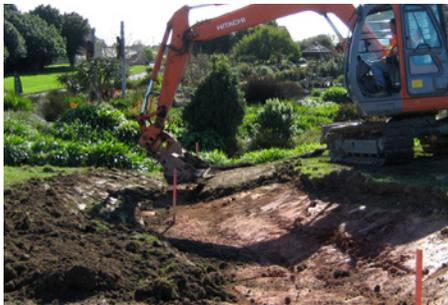
Fig.7 Preparation of top soil layer (minimum 100mm) for planting
