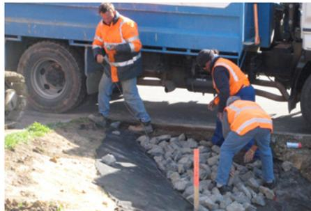
Fig.6 Construction of inlets with erosion protection
