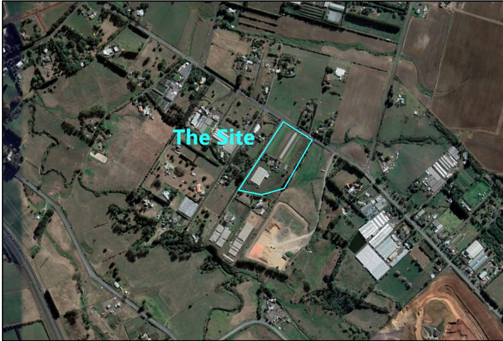
June 2022 – The site remains largely unchanged. Earthworks are underway on land to the south of the site.
