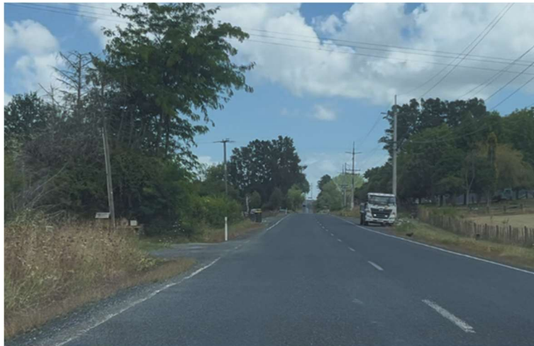
Figure 3: Fitzgerald Road near subject site (view towards north)
