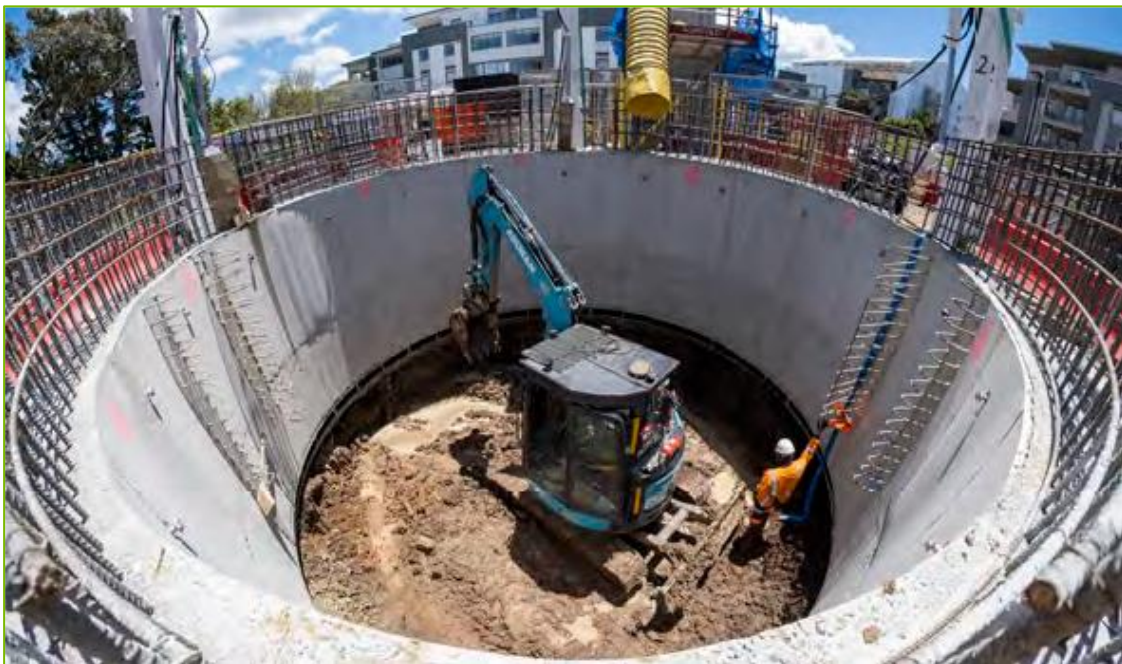
Figure 7 Cast In-situ Caisson Excavation – Central Interceptor
