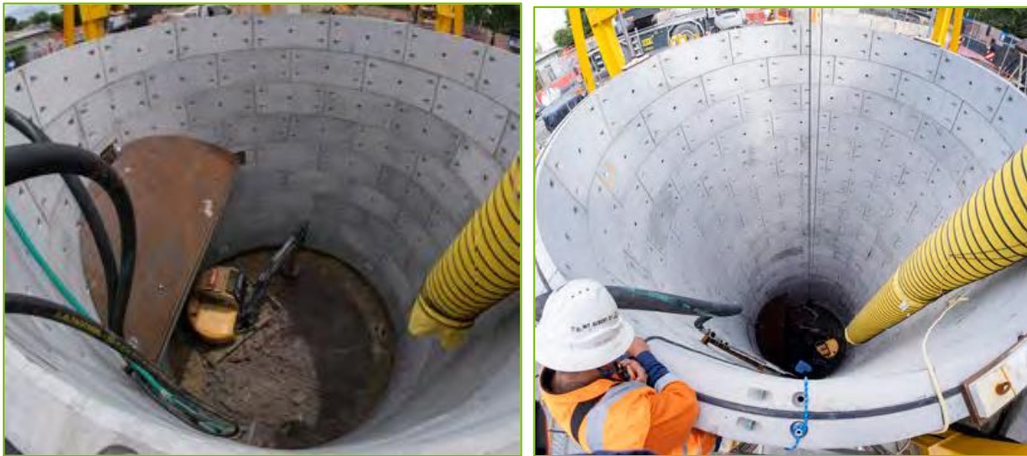
Figure 6 Pre-cast Segmental Concrete Caisson Excavation – Central Interceptor
