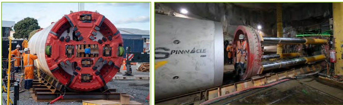
Figure 8 Micro-tunnelling (pipe jacking machine) and jacking pipe – Central Interceptor
