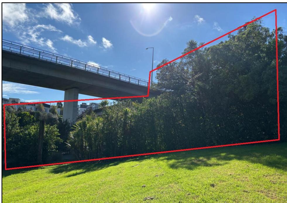
Figure 4: Vegetation removal (outlined in red) necessary to enable access and facilitate construction of Shaft 2.
