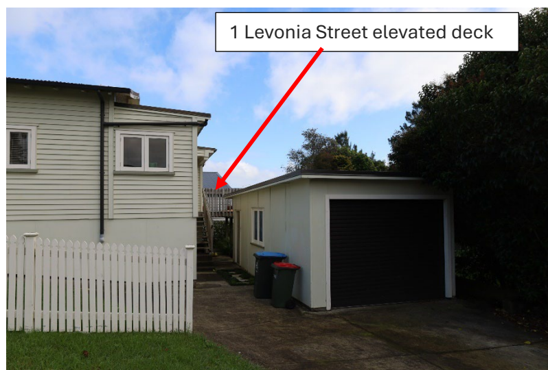
Photograph 13: Side access to 1 Levonia Street and elevated deck
