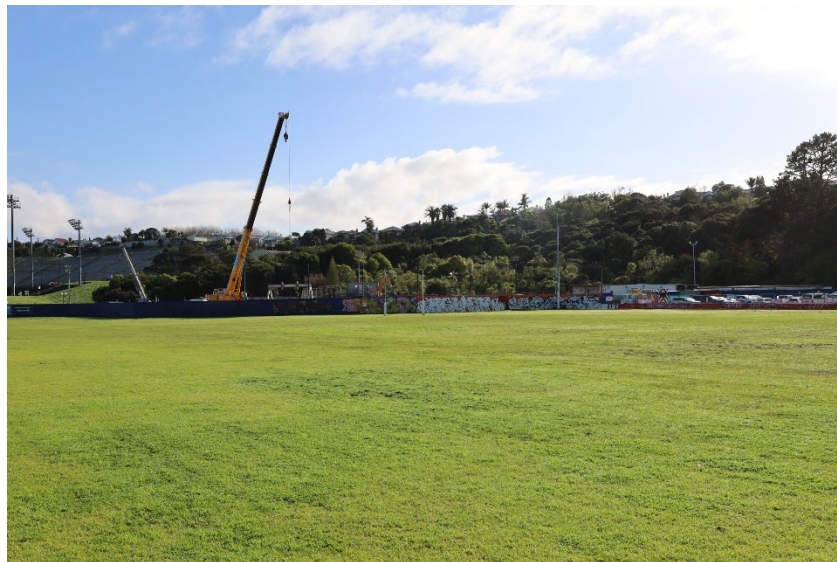
Photograph 18: Established site compound for SH08 in Western Springs Park.
