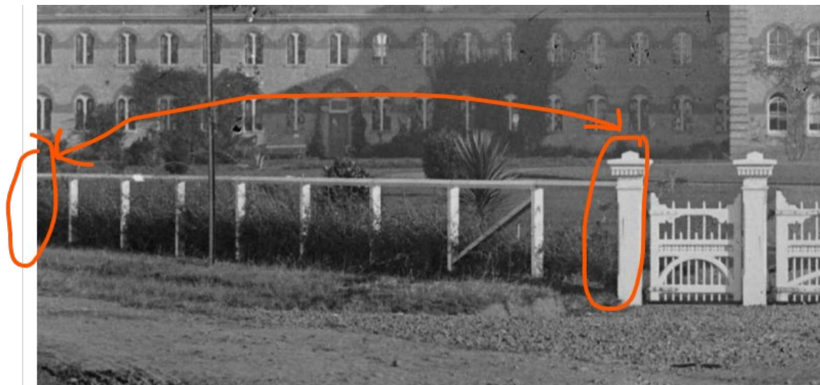
DETAIL VIEW OF BOUNDARY FENCE, SHOWING TIMBER POSTS, RAILS, WIRES AND HEDGING
