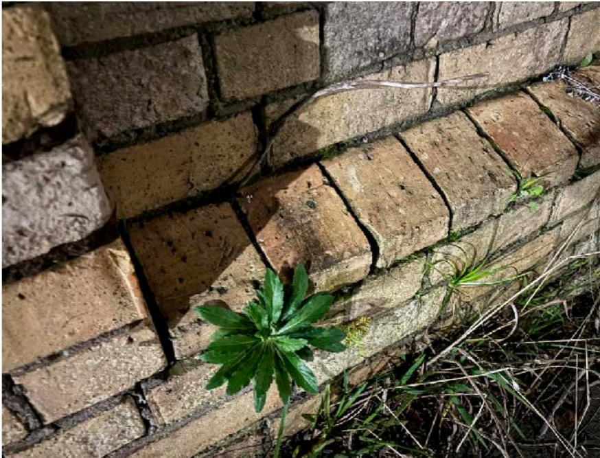
ANGLED BRICK STRING COURSE AT BASE OF WALL PANELS
