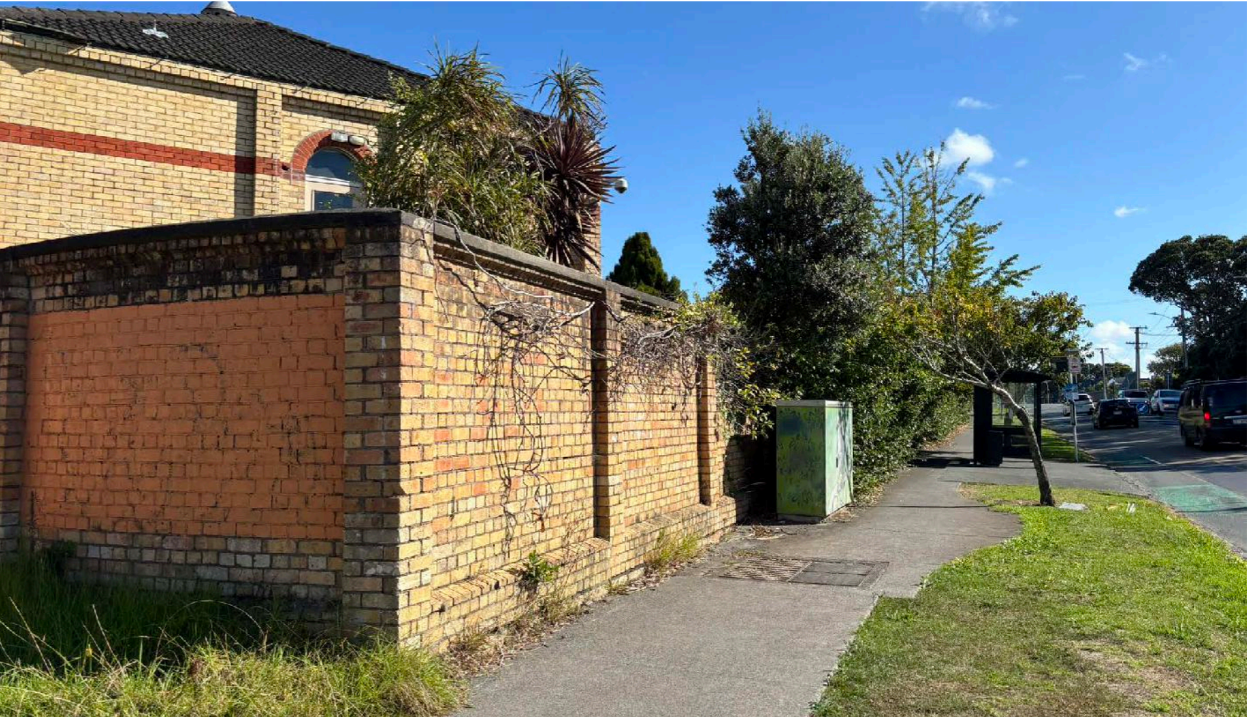
BRICK WALL CONDITION 2024, SHOWING RECTANGULAR INSET PANELS, PILASTERS RENDERED CAPPING AND VARIABLE HEIGHT WALL BASE
