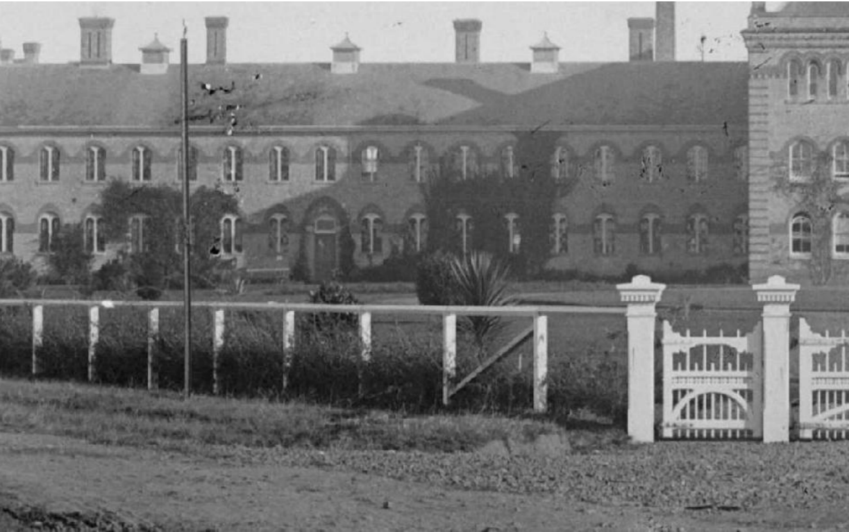
DETAIL VIEW OF BOUNDARY FENCE, SHOWING TIMBER POSTS, RAILS, WIRES AND HEDGING
