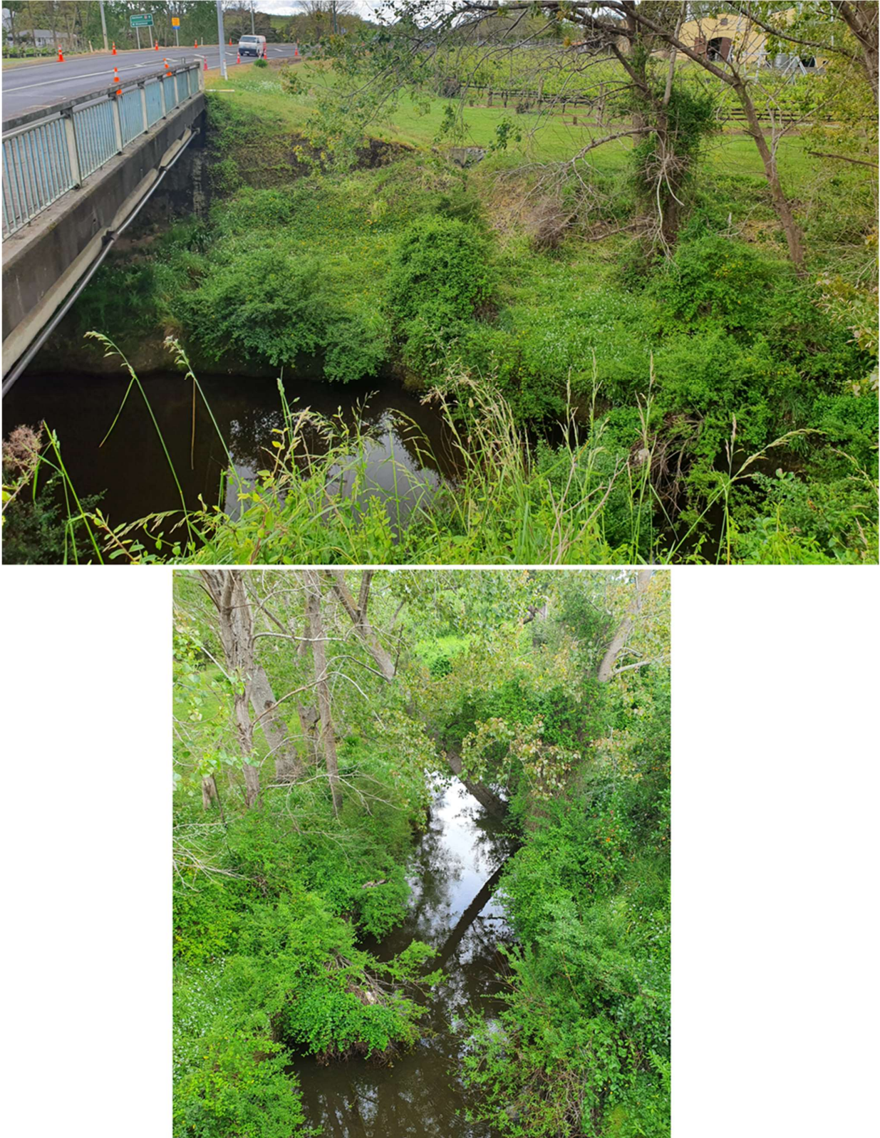
Figure 13. The Kumeū River adjacent to the SH16 bridge. Left shows the upstream section viewed from the bridge, and right shows the river viewed from the western bank (taken during the site visit on 14 th October 2020).
