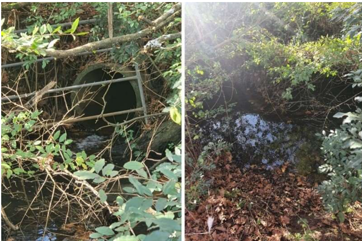
Figure 11. The culvert connecting Watercourse 4 and 3 (left) and the stream channel (right) of Watercourse 4 (taken during the site visit on 29 th June 2021).
