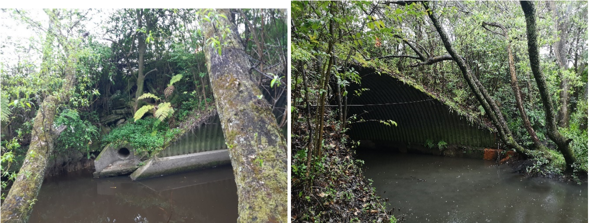
Figure 5: Existing Arch Culvert at Ngongetepara Stream. Left: Immediately upstream of the culvert looking at the true left bank with existing outfall | Right: Immediately upstream of the culvert looking at true right bank (image from October 2021).
