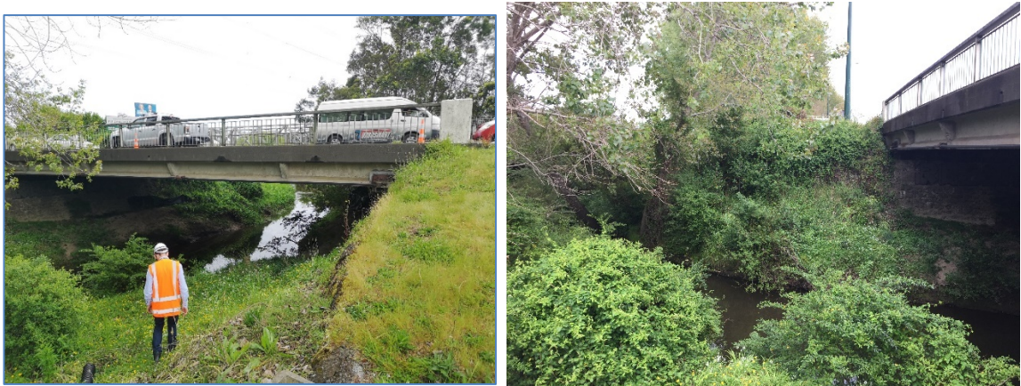
Figure 6: Existing road bridge at Kumeu River. Left: Photo taken from upstream on the true right bank, looking north | Right: Photo taken from upstream on the true right bank, looking west (image from October 2020).
