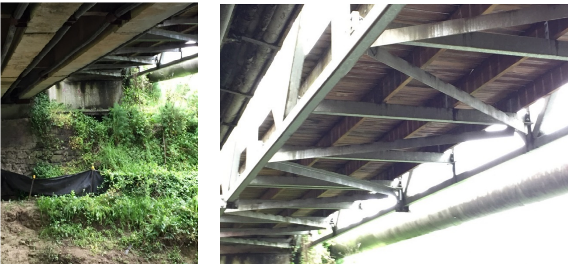
Figure 7: Existing footbridge at Kumeu River. Left: Photo of north-western bridge abutment | Right: Photo of underside of footbridge.
