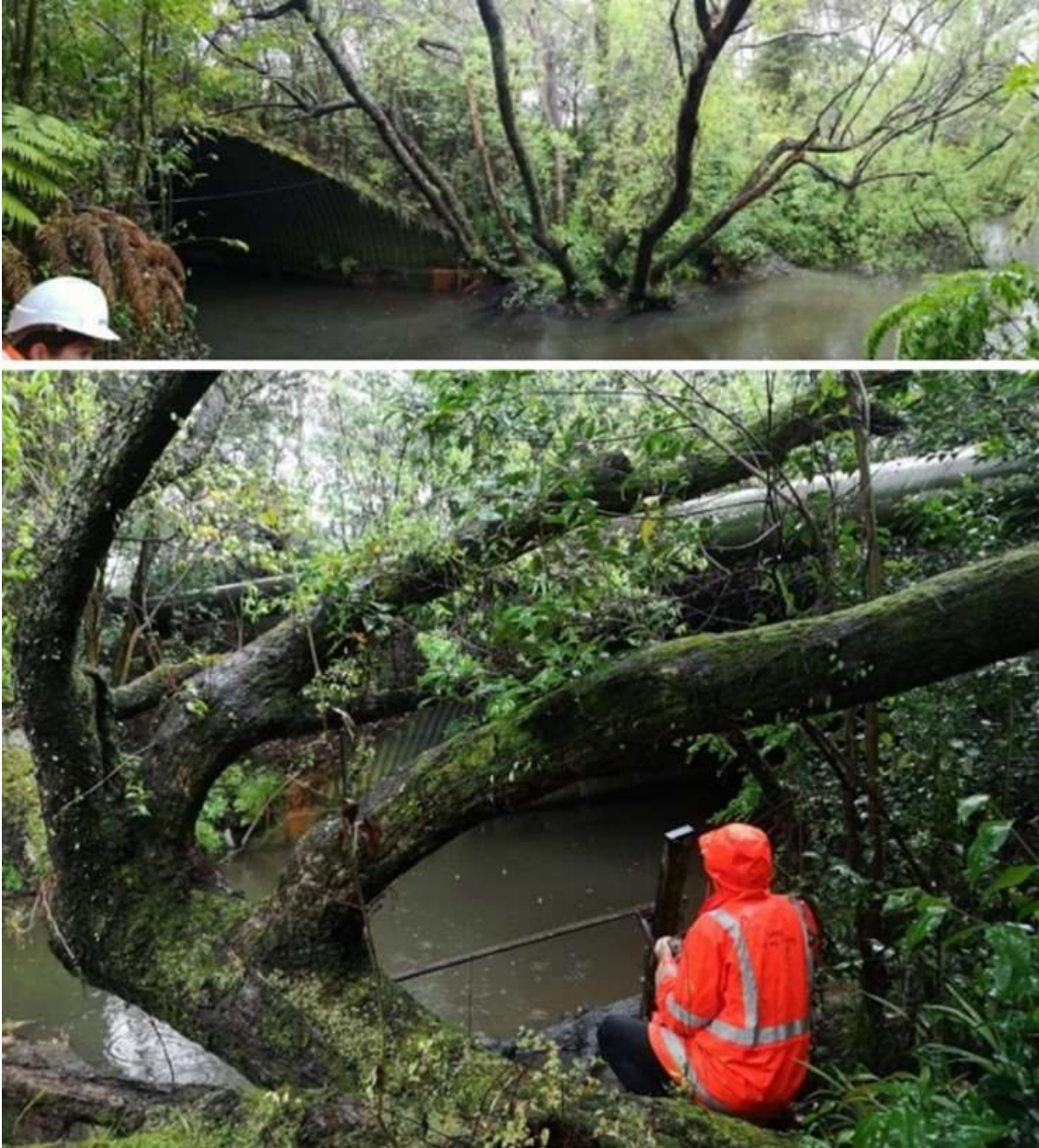
Figure 7. The southern/upstream (top) and northern/downstream (bottom) sides of the Ngongetepara Stream to the culvert.
