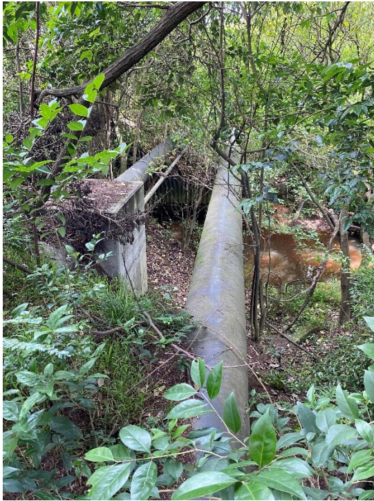
Figure 28. View facing northwest showing water pipes crossing Brigham Creek to the east of the SH16 bridge
