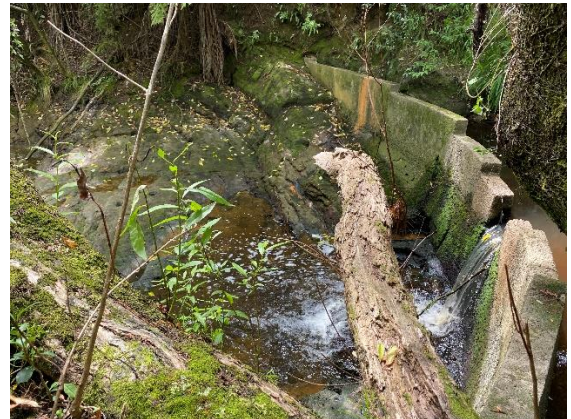
Figure 27. Concrete weir to the east of the SH16 bridge at Brigham Creek
