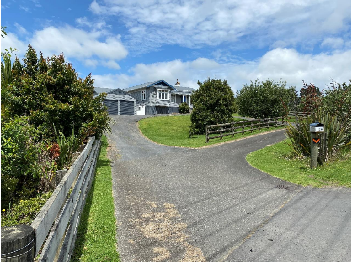
Figure 25. View facing west showing the building at 238 SH16, being the Sinton House recorded as CHI ID 13241, R11/2828 and AUP OP ID 525
