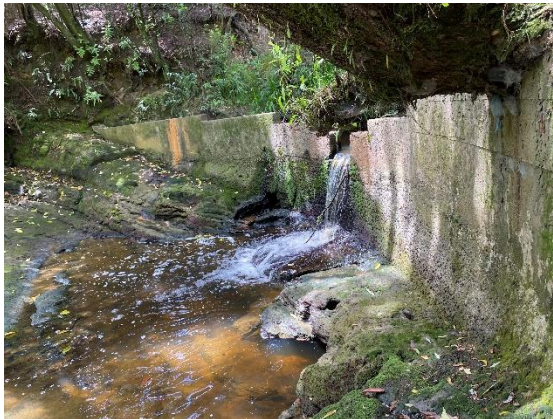
Figure 26. Concrete weir to the east of the SH16 bridge at Brigham Creek
