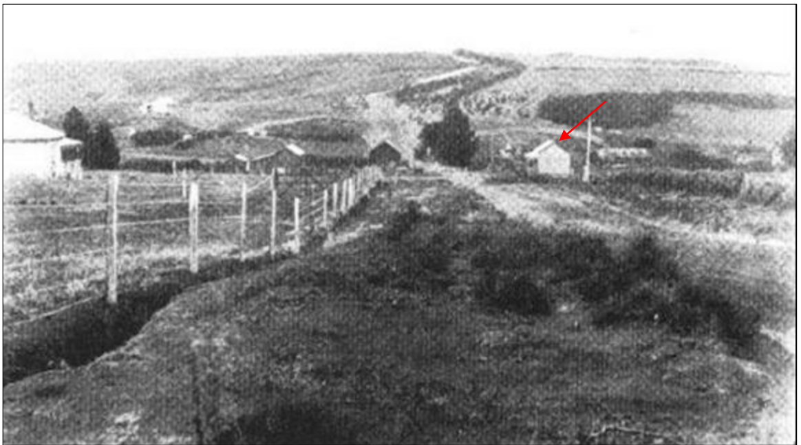
Figure 7. Looking northwest from eastern side of creek c.1902, showing Alex Sinton's house (222a SH16, left), John Sinton's original house (left background), the Store (arrowed) and beyond it the original house and picket fence on the western side of the creek (from Madden 1966: 122)
