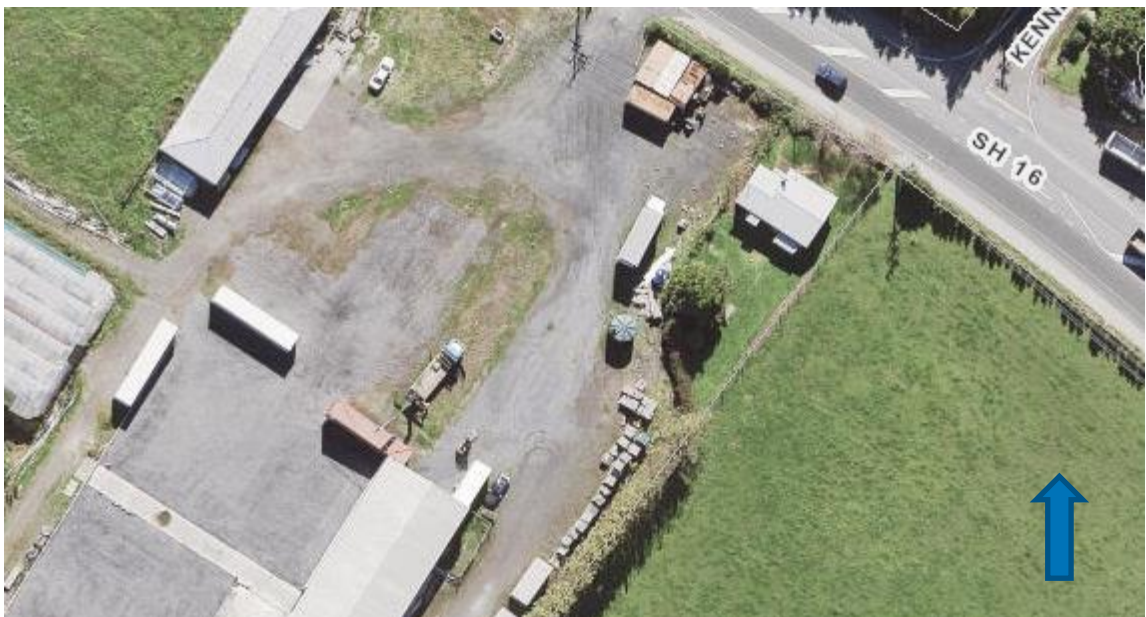
Figure 9: Assessment area West 1 – Aerial photo
