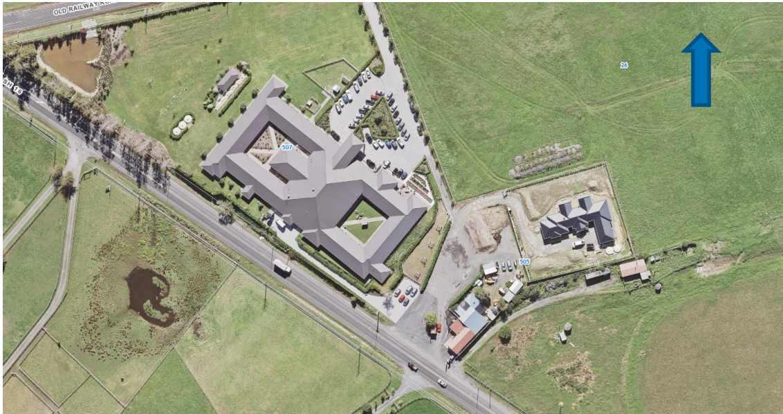
Figure 8: Assessment area East 9 – Aerial photo
