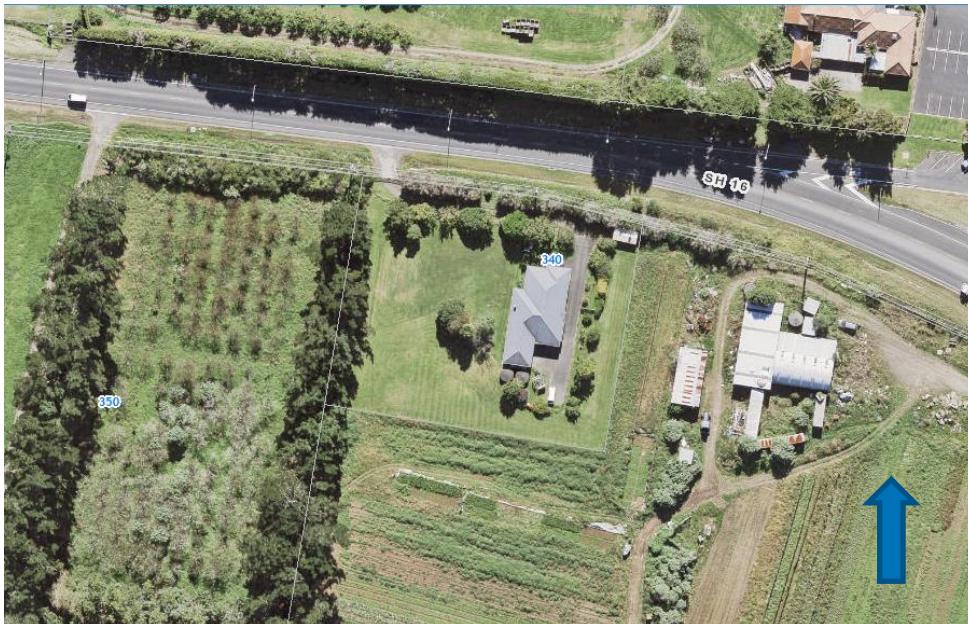
Figure 13: Assessment area West 5 – Aerial photo
