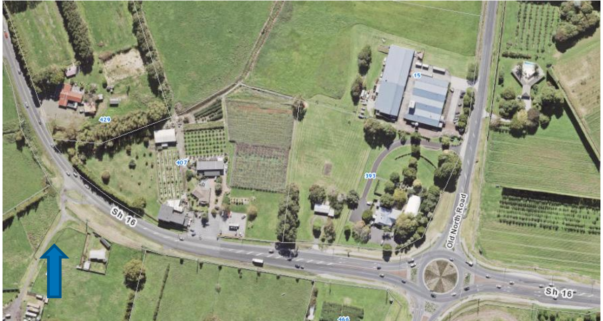
Figure 5: Assessment area East 6 – Aerial photo
