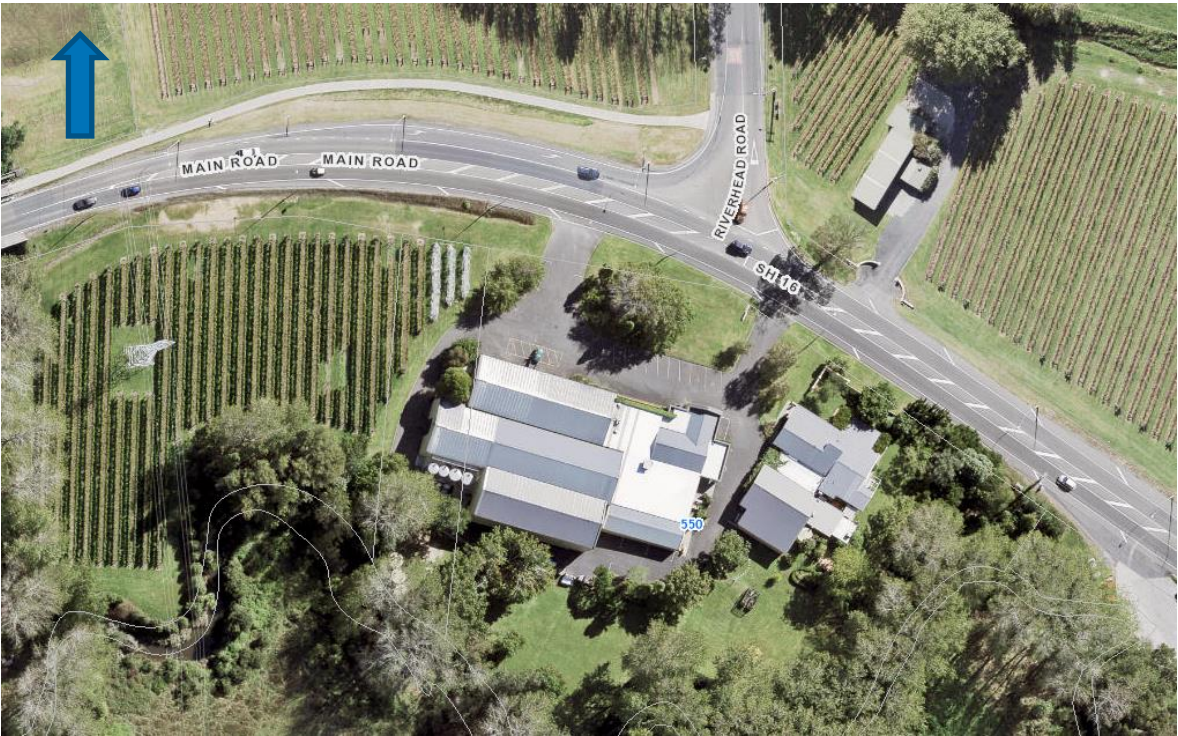
Figure 15: Assessment area West 7 – Aerial photo
