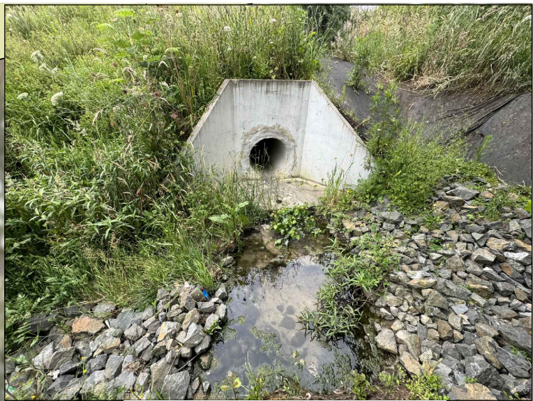
STORMWATER OUTLET - PHOTO 1
