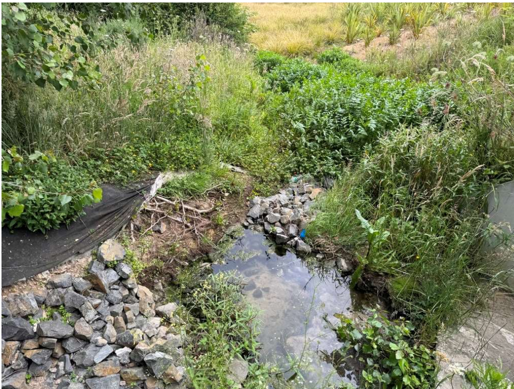
Image 4: Existing riprap apron (28 November 2023)
