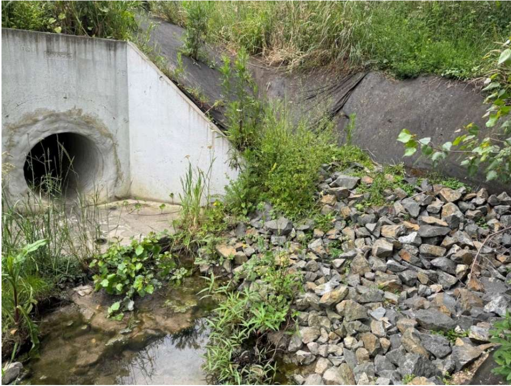
Image 3: Existing wingwall outlet (28 November 2023)
