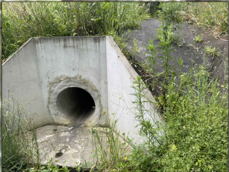
STORMWATER OUTLET - PHOTO 2
