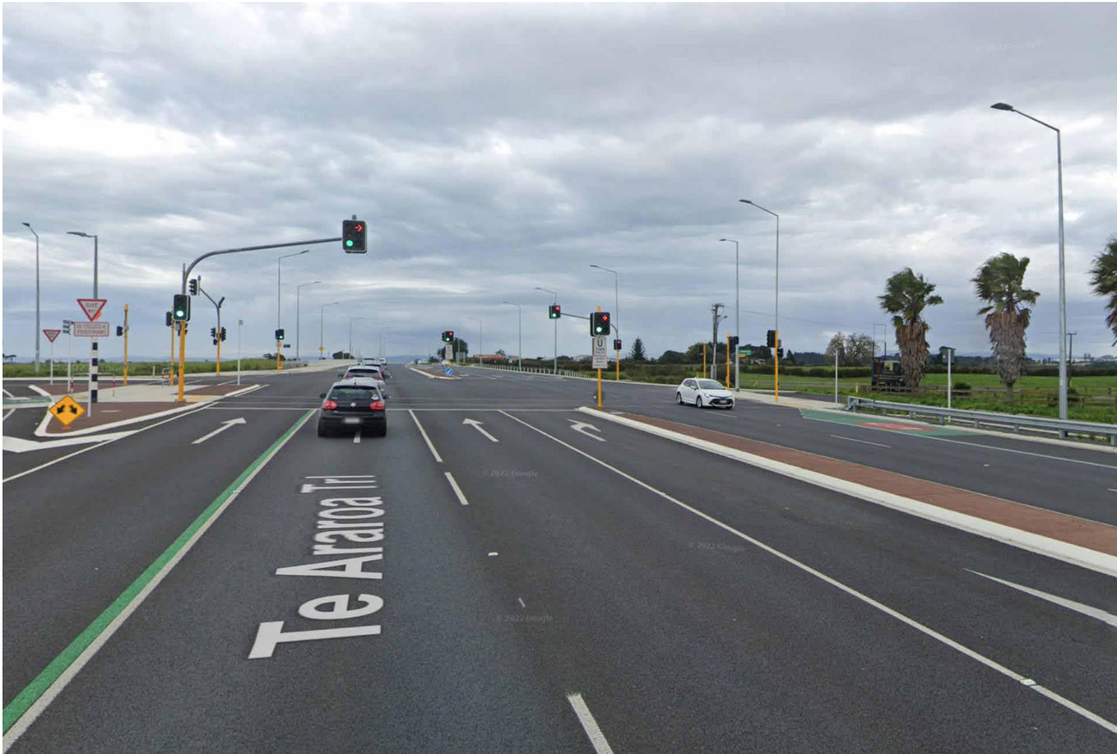
2. LOOKING SOUTH-WEST TOWARDS THE AIRPORT JUNCTION AT PUHINUI RD & CAMPANA RD
