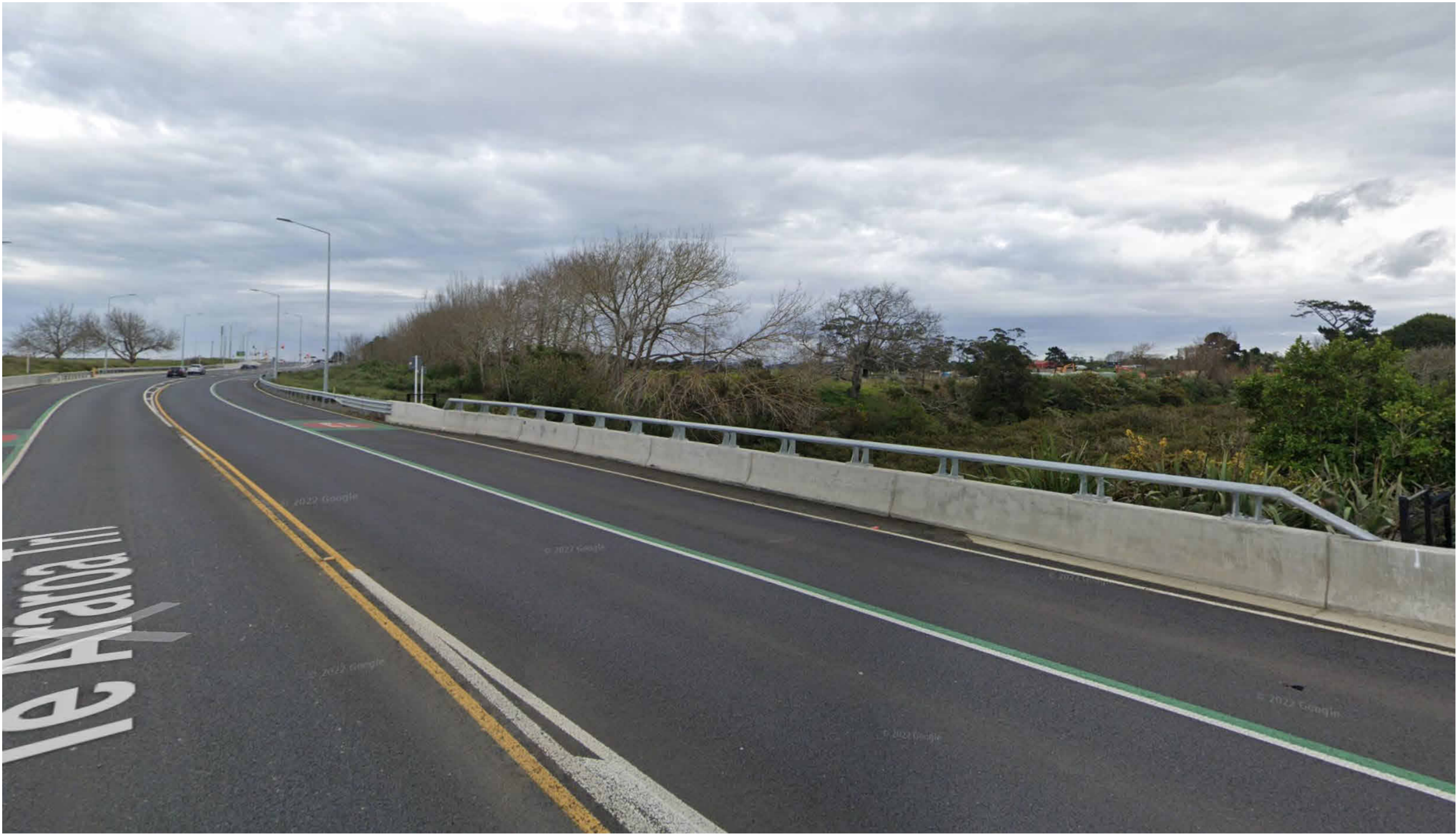
1. LOOKING WEST TOWARDS THE SITE
