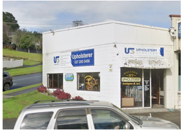
Figure 12: 87 Commercial Road (Google Street View, July 2020)
