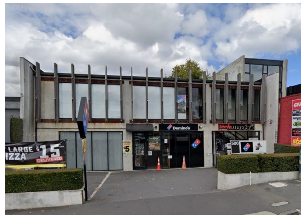
Figure 10: 498 New North Road (Google Street View, March 2021)
