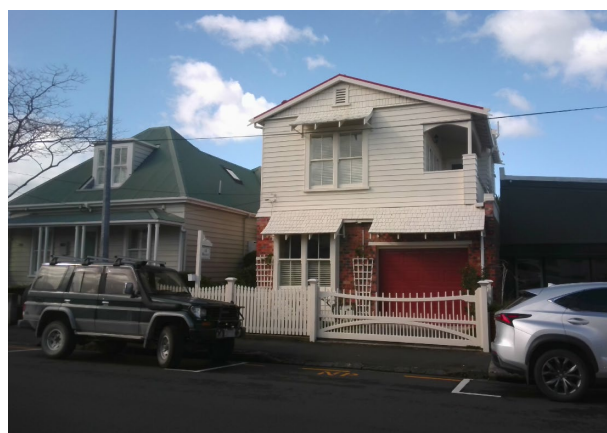
Figure 6: 14 and 16 Wynyard Street
