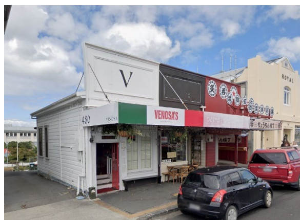
Figure 6: 480-484 New North Road (Google Street View, March 2021)
