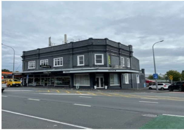
Figure 3: Owen's Buildings, 215 Dominion Road
