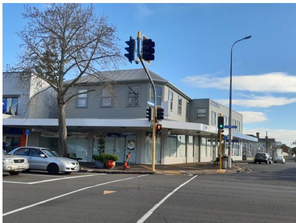
Figure 11: Arch Hill Hotel (former), 584 Great North Road
