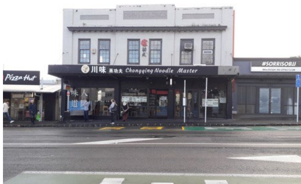
Figure 1: Owen's Buildings, 191-217 (215) Dominion Road
