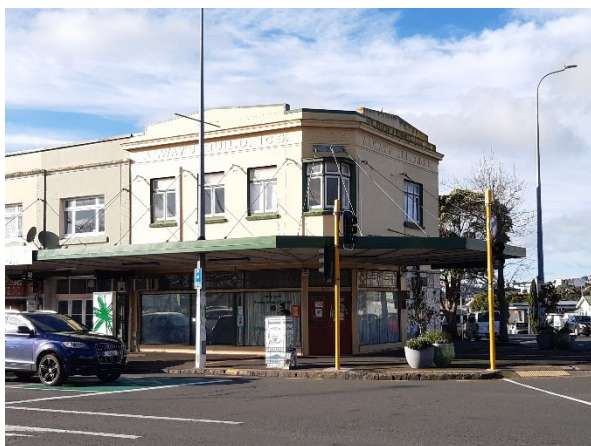
Figure 1: Alway's Buildings, 543 Great North Road
