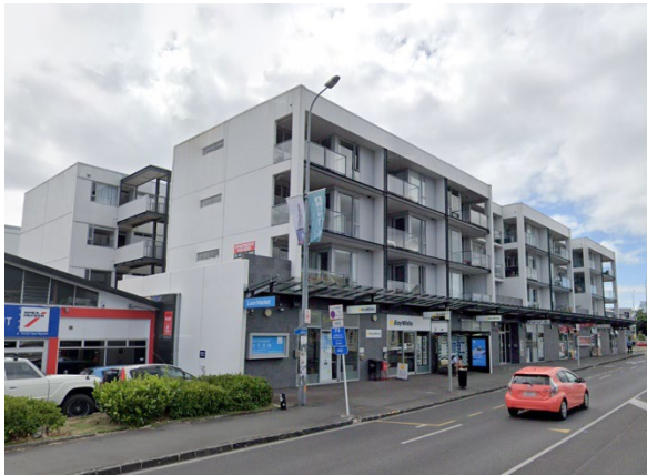
Figure 7: 433-437 New North Road (Google Street View, March 2021)
