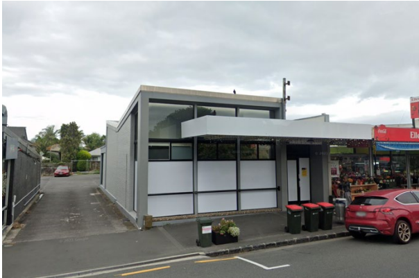
Figure 7: 133A Main Highway (Google Street View, March 2021)
