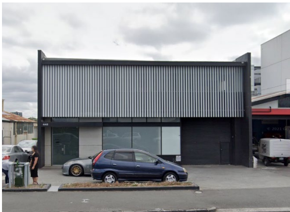
Figure 9: 445 New North Road (Google Street View, March 2021)
