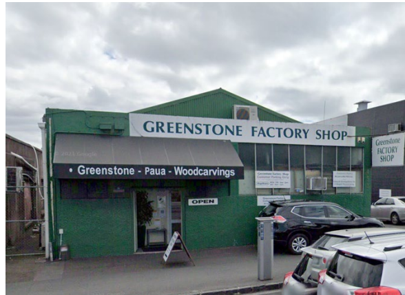
Figure 8: 453 New North Road (Google Street View, March 2021)
