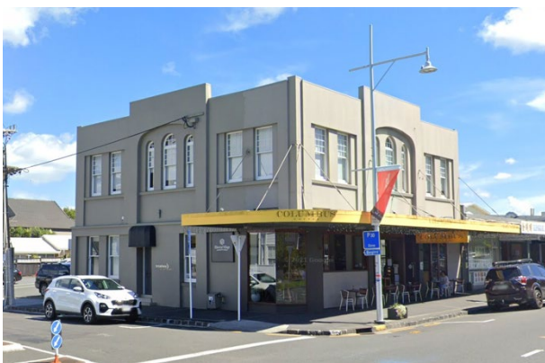
Figure 1: Former Borough Council Chambers, 137-141 Main Highway (Google Street View, March 2021)
