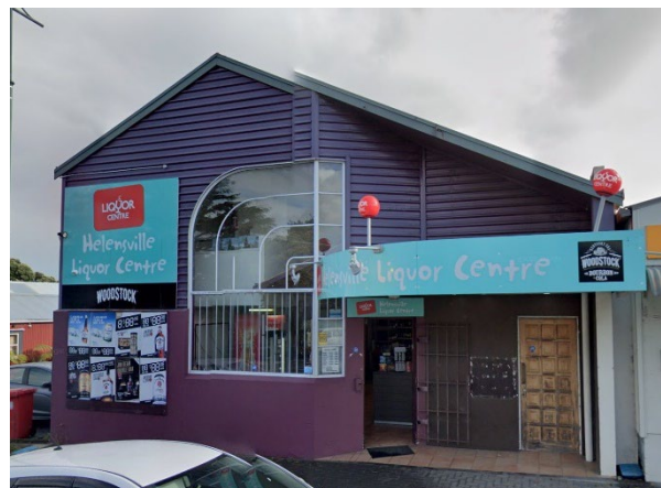
Figure 10: 88 Commercial Road (Google Street View, July 2020)
