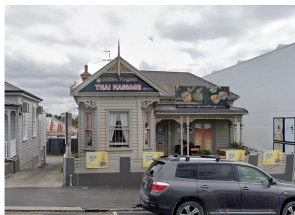
Figure 5: 511 New North Road (Google Street View, March 2021)
