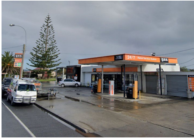
Figure 11: 4-16 Railway Street (Google Street View, July 2020)
