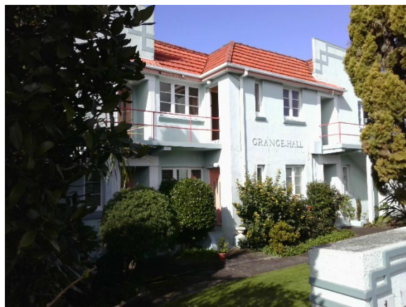
Figure 4: Grange Hall Apartments, 492 Mount Eden Road
