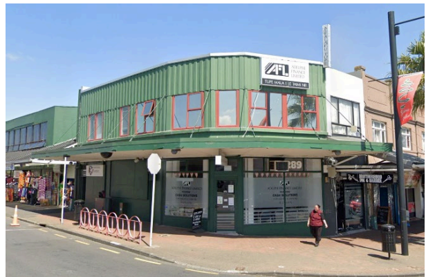
Figure 10: 289 Great South Road (Google Street View, August 2020)
