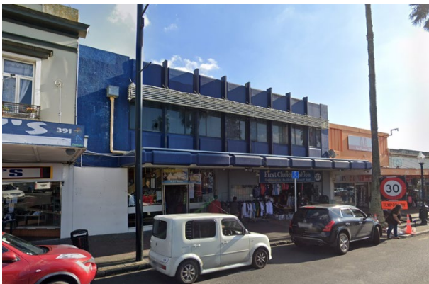
Figure 9: 387 Great South Road (Google Street View, August 2020)
