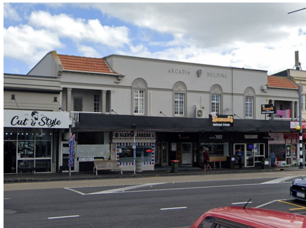
Figure 2: Arcadia building, 521-531 Sandringham Road (Google Street View, March 2021)
