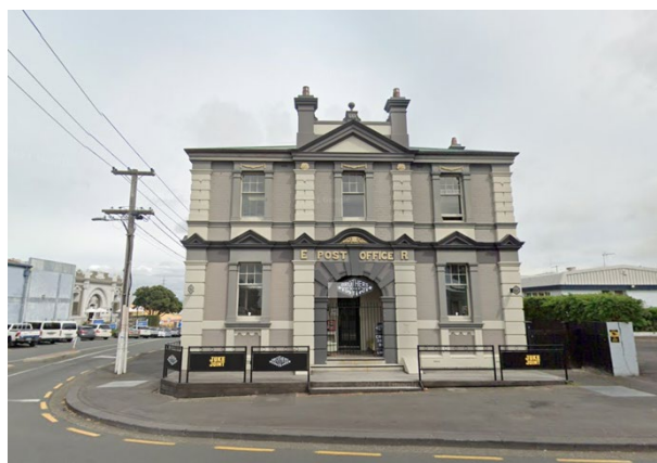
Figure 2: Post Office (former), 120 Onehunga Mall (Google Street View, March 2021)
