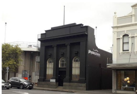
Figure 4: Former ASB Bank, 29 Khyber Pass Road
