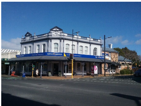
Figure 1: Till and Son Building, 427-429 Mount Eden Road
