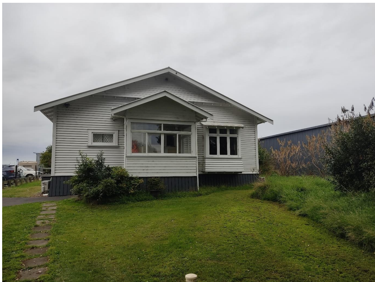
Figure 19: Building "C" (see map above), a bungalow from possibly the 1920s or 1930s with substantial later additions and renovations.
