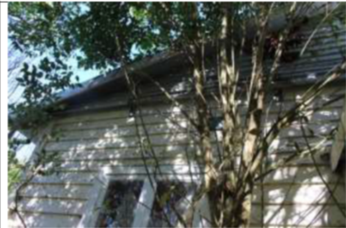
N (rear) elevation looking S
