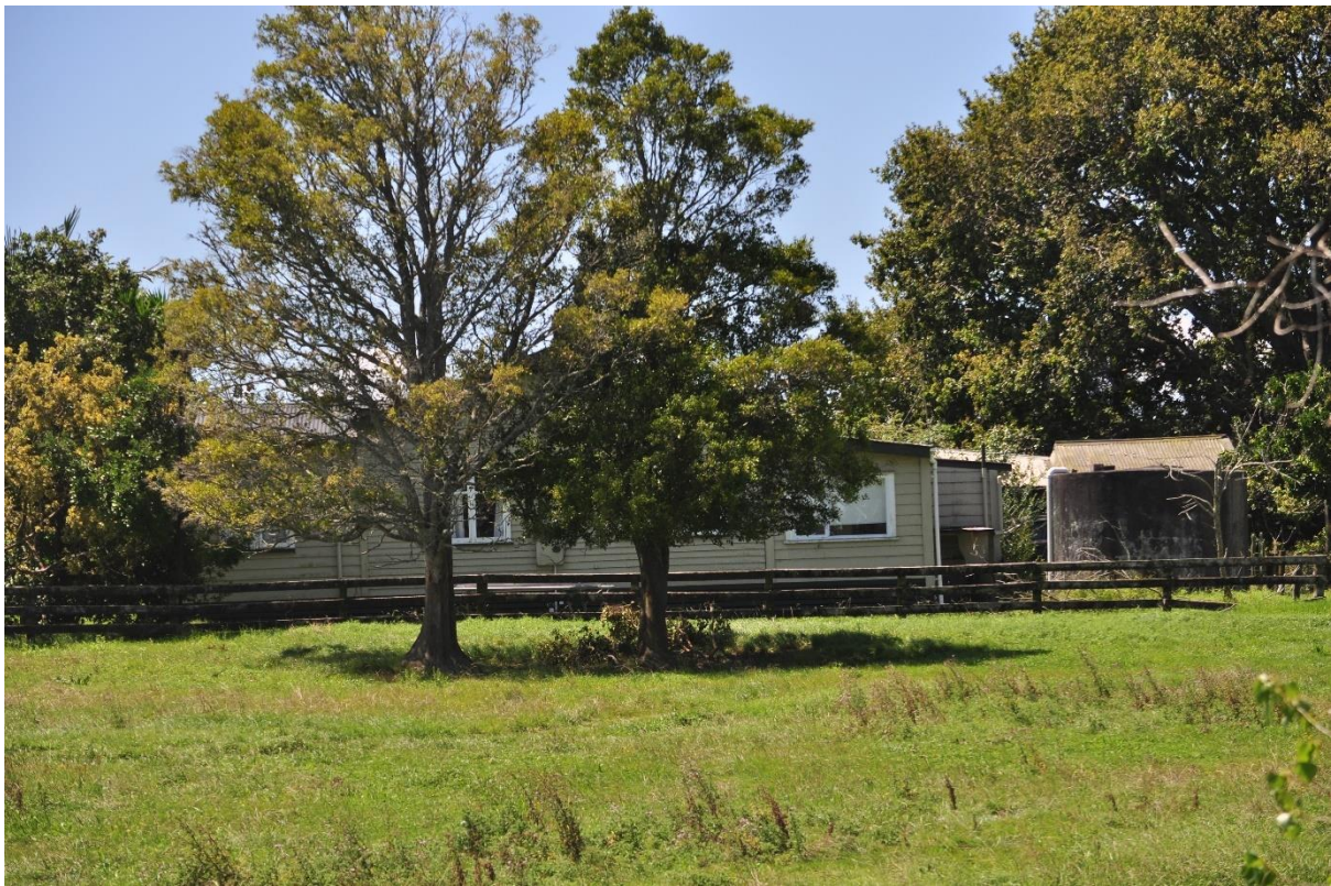
Figure 17: Second 1930 - 40 (?) farm building.
