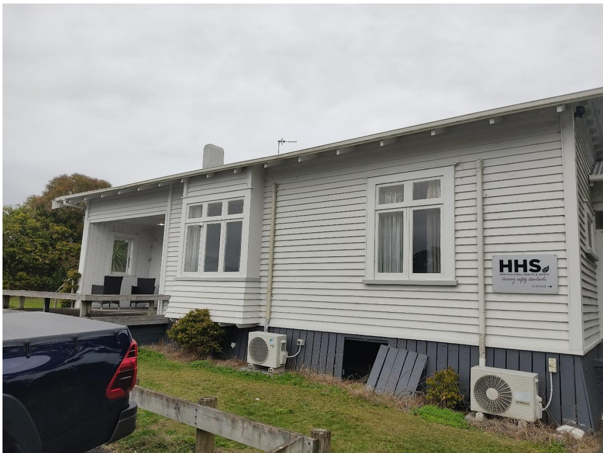
Figure 24: Bungalow style building "C", probably built in the 1920s or 1930s. Veranda on the left is a later addition.
