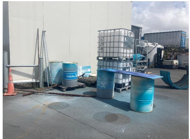
Photo 14: Spray painting area on western side of workshop
