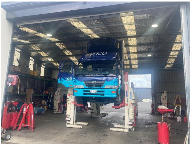
Photo 11: View looking east at the main hoist.
