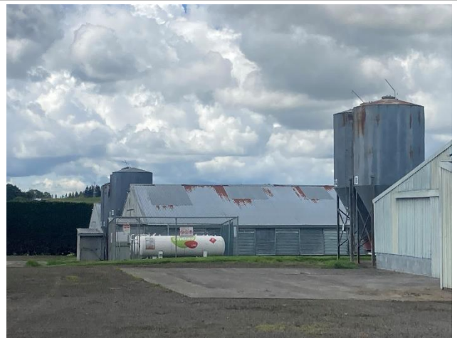
Photo 33: Grain silos and LPG containers at the eastern end of the poultry sheds
