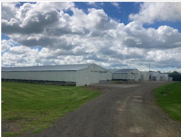
Photo 32: Poultry sheds at 370 Karaka Road
