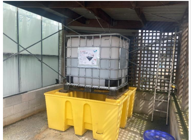
Photo 27: Nitric acid storage. The concrete showed some evidence of acid etching.
