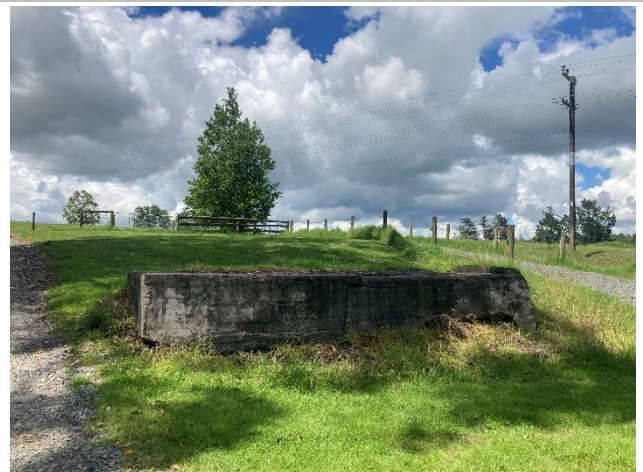
Photo 41: Concrete base of former shed
