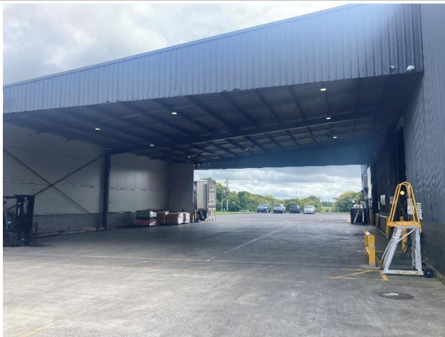
Photo 1: Loading bay at the packing and distribution building
