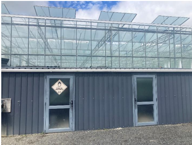
Photo 26: Water pump shed and chemical storage.
