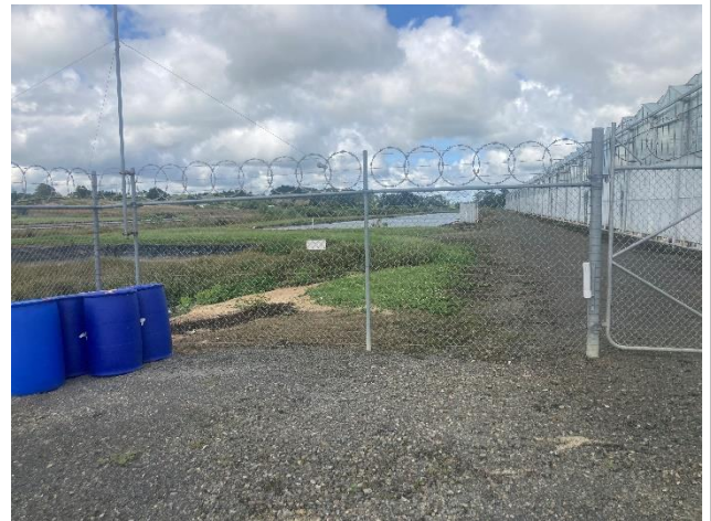
Photo 29: Effluent ponds. The first pond is visible behind the blue barrels, with the second (larger) pond in the distance.
