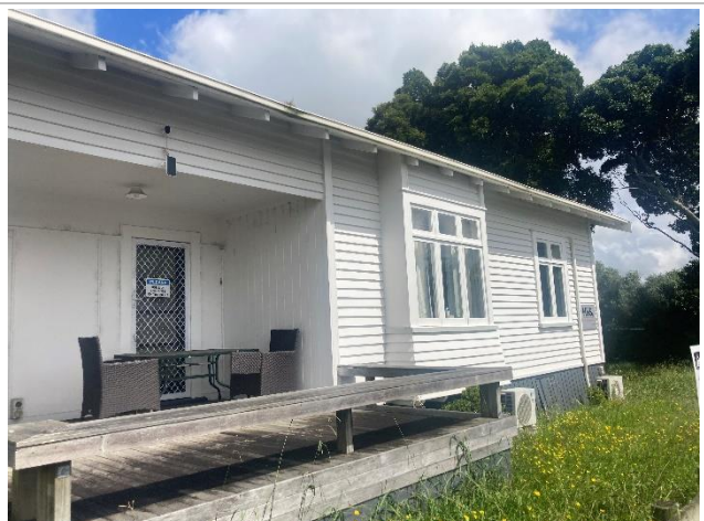
Photo 4: House at 300 Karaka Rd. Suspected ACM panels are visible to the left of the photo. Paint is in excellent condition.
