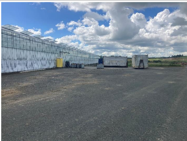
Photo 30: Storage area at the southwest side of the glasshouses. Waste plant materials are at the rear right.
