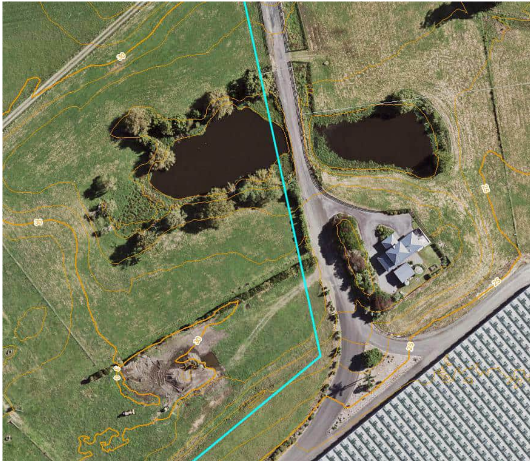
Figure 3: Pond in south-east corner of #350. Note the topsoil stockpile works. (2017 Aerial Photo with 1.0m contours from Auckland Council GIS).
