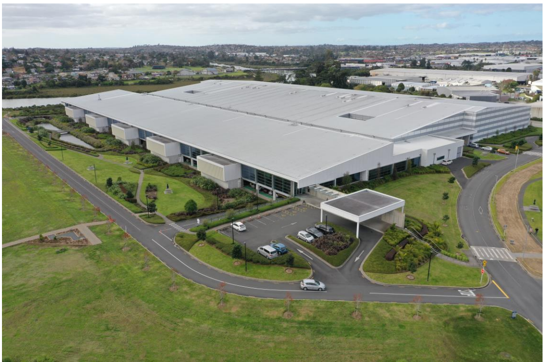
Figure 2 Photograph of the Daniell Building at the existing East Tāmaki Fisher & Paykel Healthcare Campus
