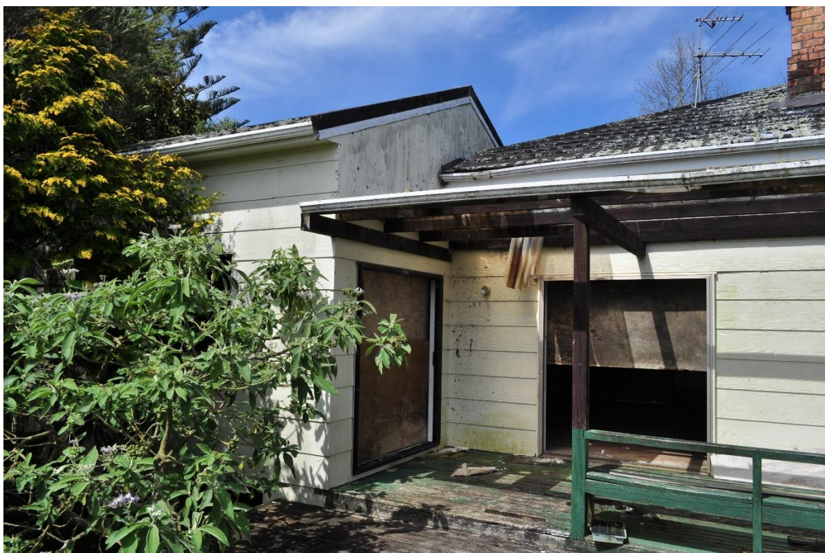
Figure 18: Northern side of the house.
