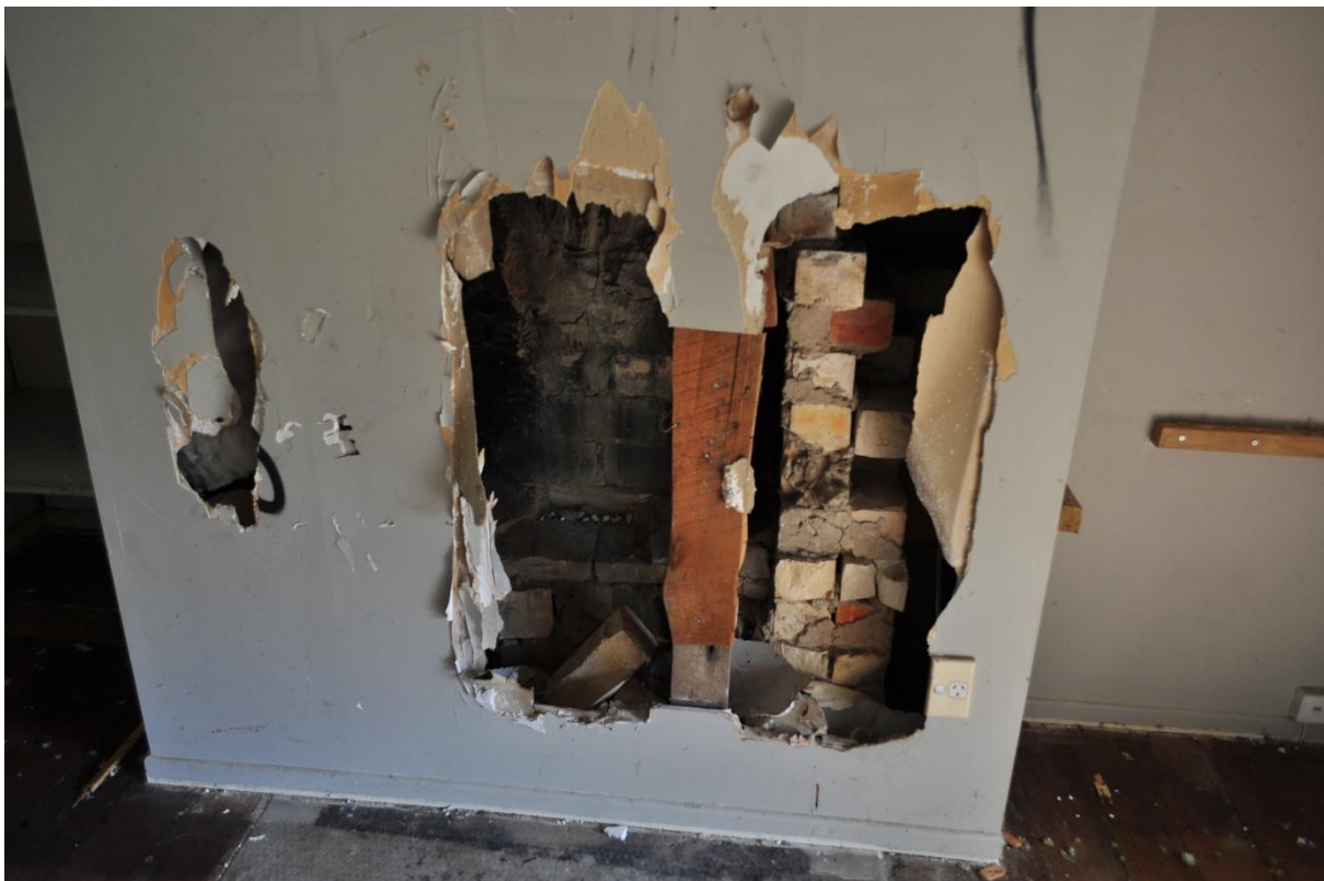
Figure 17: Renovations plastered over the original fireplace.
