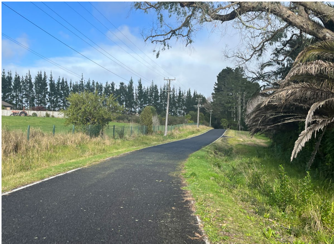
Rural road formation at Sinton Road (7 Sinton Road on left hand side)
