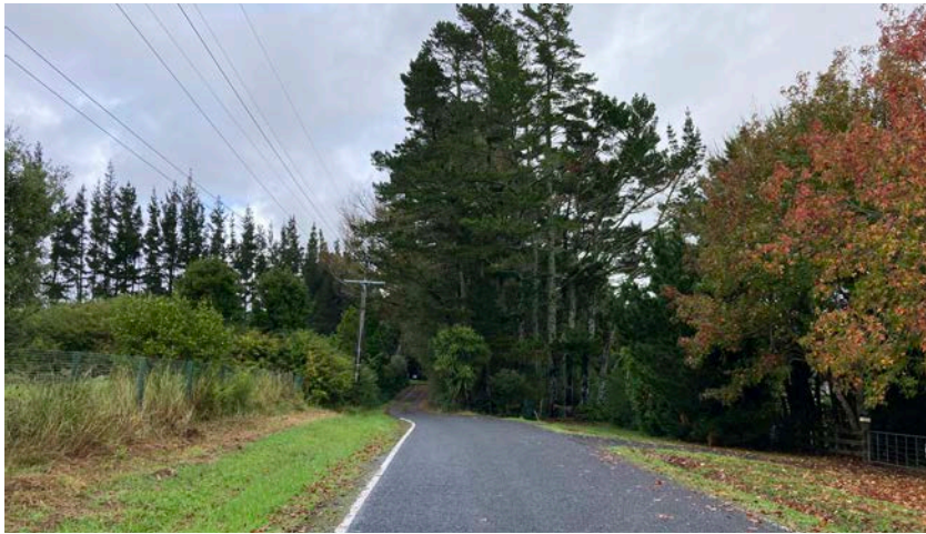
2. Looking towards the western 'Paper Road' end of Sinton Road.
