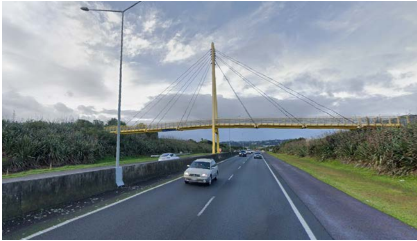
6. The Clarks Lane footbridge, which links the northern half of the Neighbourhood Plan Area with Hobsonville Local Centre over SH18.
