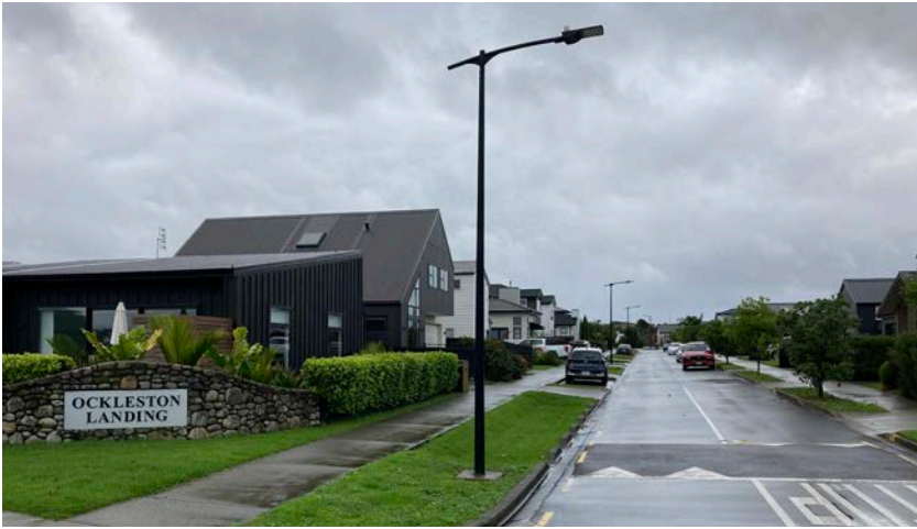
5. A residential street within the Ockleston Landing subdivision.
