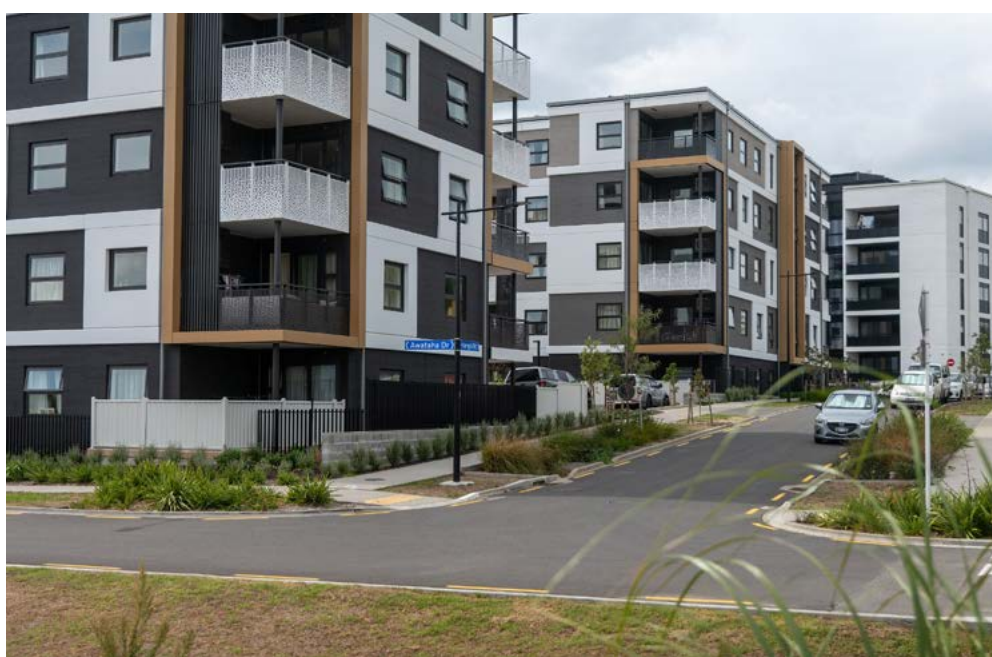
▲ New housing in Northcote
