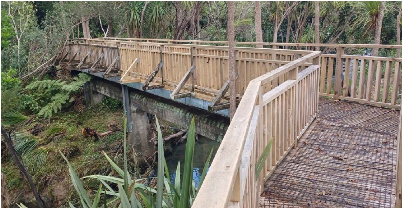
▲ The repaired Waterview Downs Bridge
