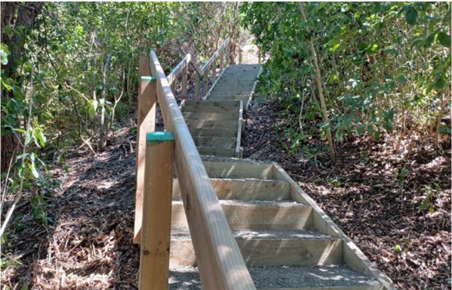
◀ New tracks as part of the Waikōwhai Coastal track upgrades
