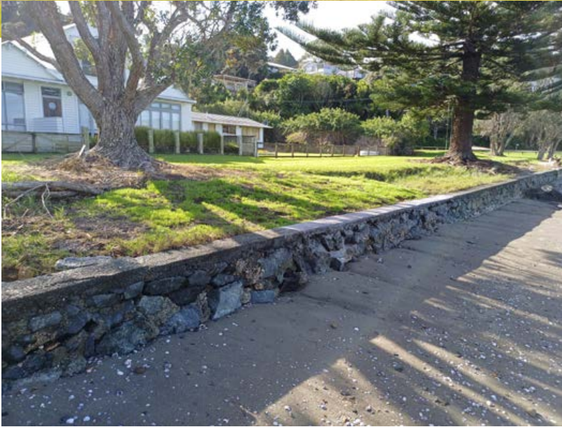
▲ The seawall at Baddeleys Beach has been repaired after storm damage.
