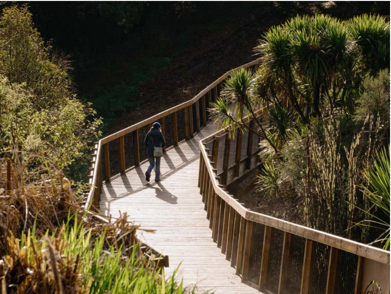
▲ The step-free footbridge at Kōwhai Park makes it easy for cyclists and walkers to access buses, nature and sports activities.
