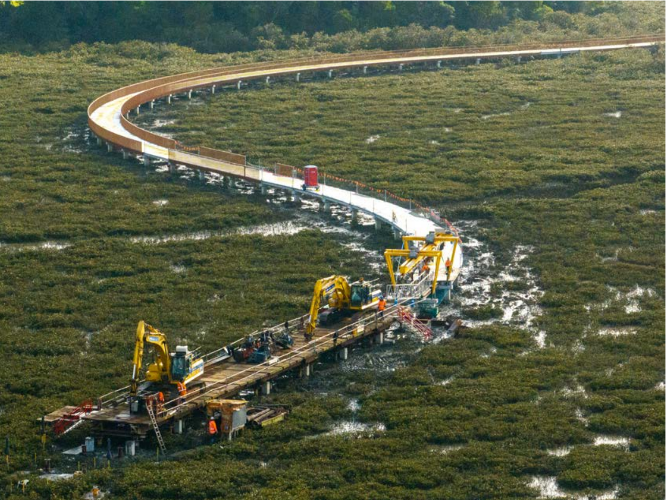
▼ Te Whau Pathway under construction
