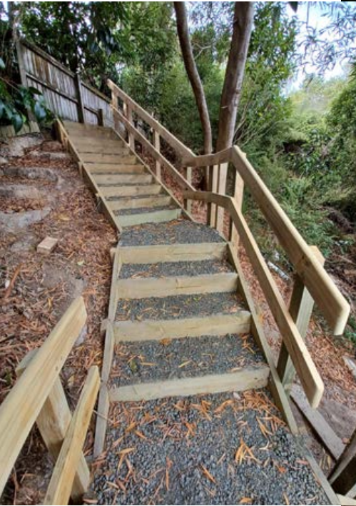
▼ Track upgrades at Bushglen Reserve include new boardwalks, stairs, handrails and a small bridge to improve access to the reserve.
